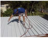
Top Picture: Rustshield W being sprayed over Galvanised metal roofing
