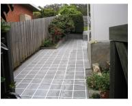
Top Picture: Stencilshield Primer Plus applied to prepared concrete.
