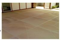
Notes Cont'd: The application of one or more splatters or shadows of colour can be sprayed using the product called Fleck Coat. This is normally applied prior to the removal of the pattern and is available in a range of colours in 4 litre pails
