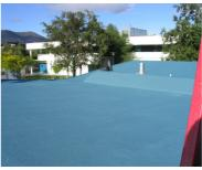
Top Picture: Poly cloth and Watershield A applied to prepared concrete. Bottom Picture: Finished Watershield A concrete rooftop.
